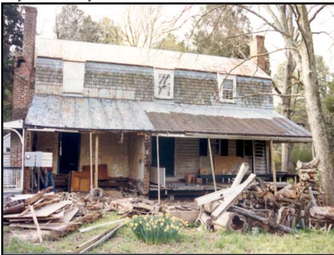
Rear view, during the Snyder Renovations, early 1989.
